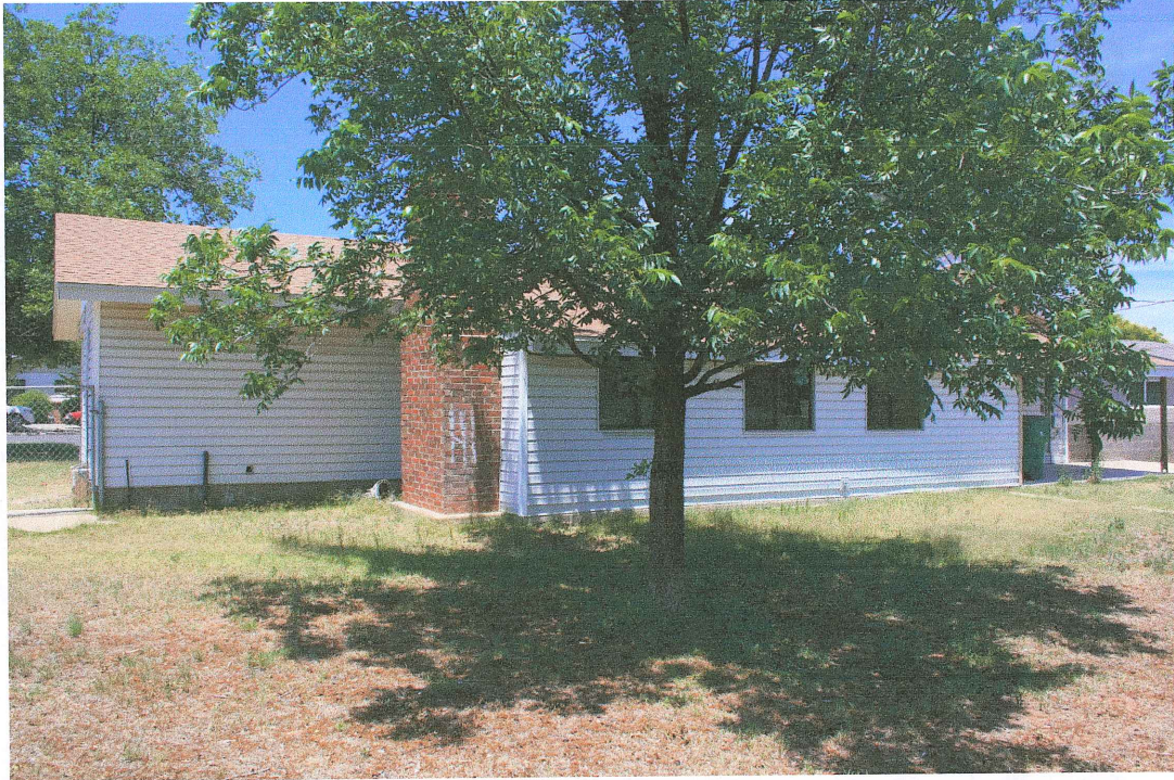
06/06/2016 SW Rear View
