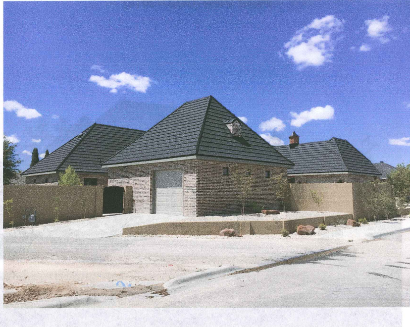
Partial Rear View (04/07/2016)
