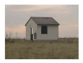
A third type of off-site facility was the radio range. This transmitter radiated coded signals in all directions in order for the aircraft to determine their bearings. It was located three miles due north of the north-south runway (Figure 20).
