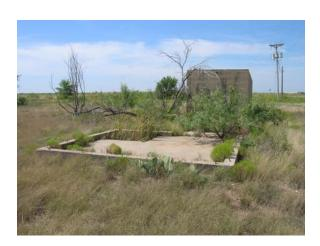
The rectangular foundation of a small boiler house is located to Building 205 (Figure 110). It features a rectangular subterranean concrete-lined pit in its southwest corner. According to historic documents it is said to have provided heat for Building 205 (TL 2005: Appendix B).
