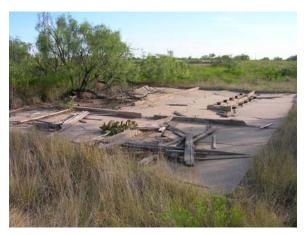
Figure 87: Building 36 concrete foundations and boards, lavatory. Note commode drains in the right center of the photograph.
