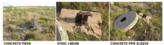
Figure 59: Features of Building 676, storehouse
