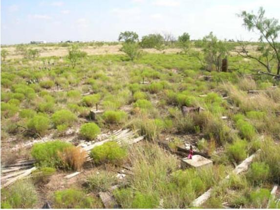
**Figure 52: Building 672 concrete piers and discarded framing lumber, hospital barracks**
