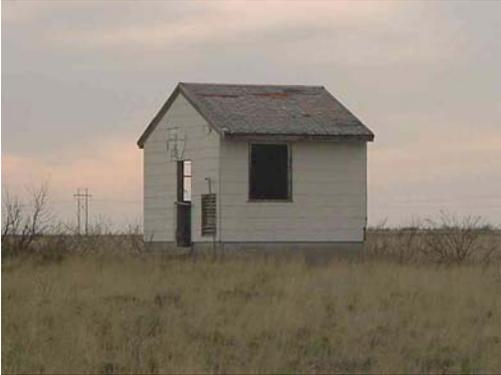
A third type of off-site facility was the radio range. This transmitter radiated coded signals in all directions in order for the aircraft to determine their bearings. It was located three miles due north of the north-south runway (Figure 20).
