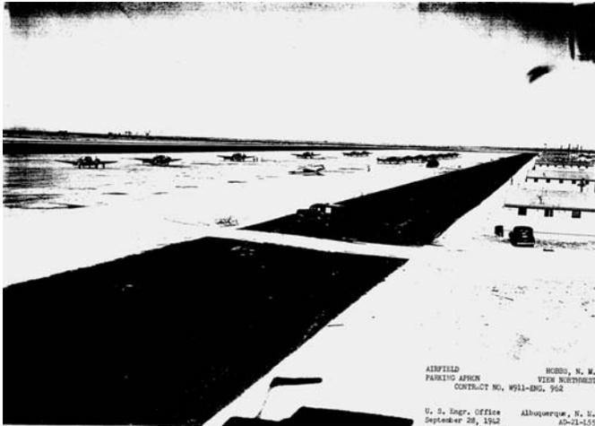
17 aircraft were pushed into the structures for regular maintenance. The parking apron or “ramp” situated directly in front of the flight line buildings was 500 feet wide and 7,600 feet long (Thole 2007: 35), and surfaced with concrete.
