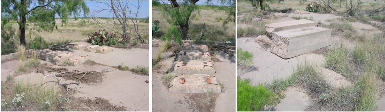
CONCRETE SLAB WITH BOILER SUPPORTS    BOILER SUPPORT DETAIL    CONCRETE POSTS
